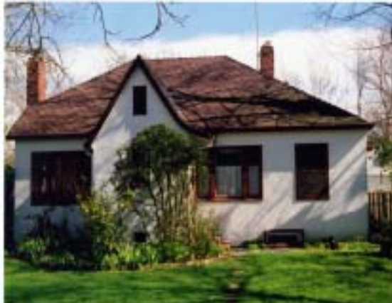
Figure 15 536 C Street English Cottage Revival
