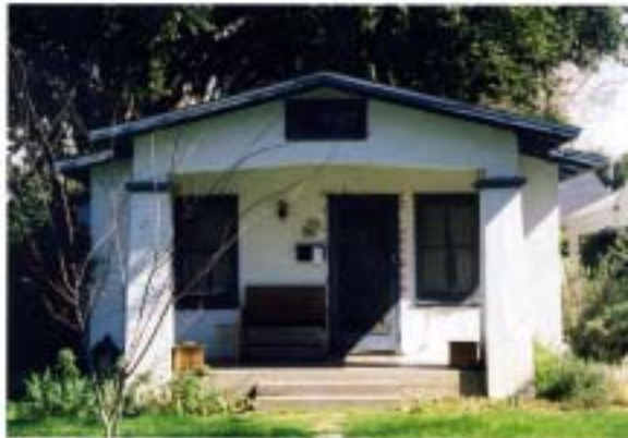
Figure 13 516 E Street Pedder Bungalow
