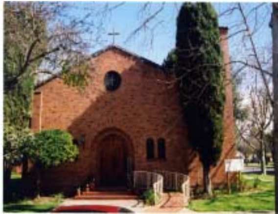
Figure 24 514 5 th Street St. James Church
