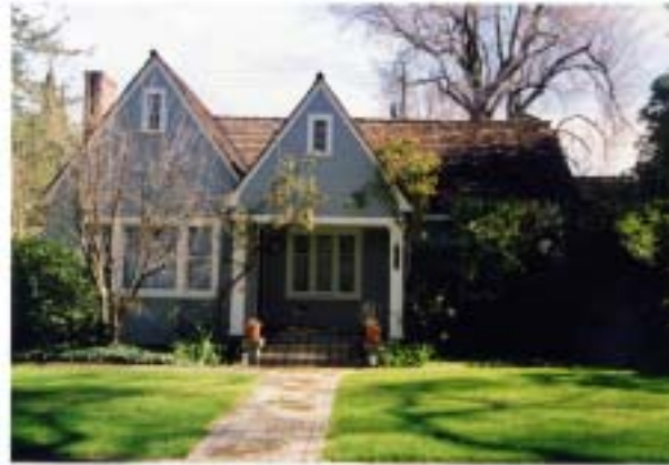
Figure 19 636 B Street English Cottage Revival
