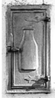
Each milk box has a small door (with no lock) that a milkman could open onto a little chamber in the wall. In it, he (yes, he) could place a quart bottle of milk. The inside wall of the box had a door that the resident could open to take out the milk.
